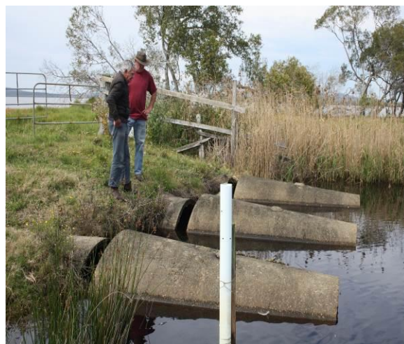
Figure 2: Poorly maintained inlets to flood gates.
